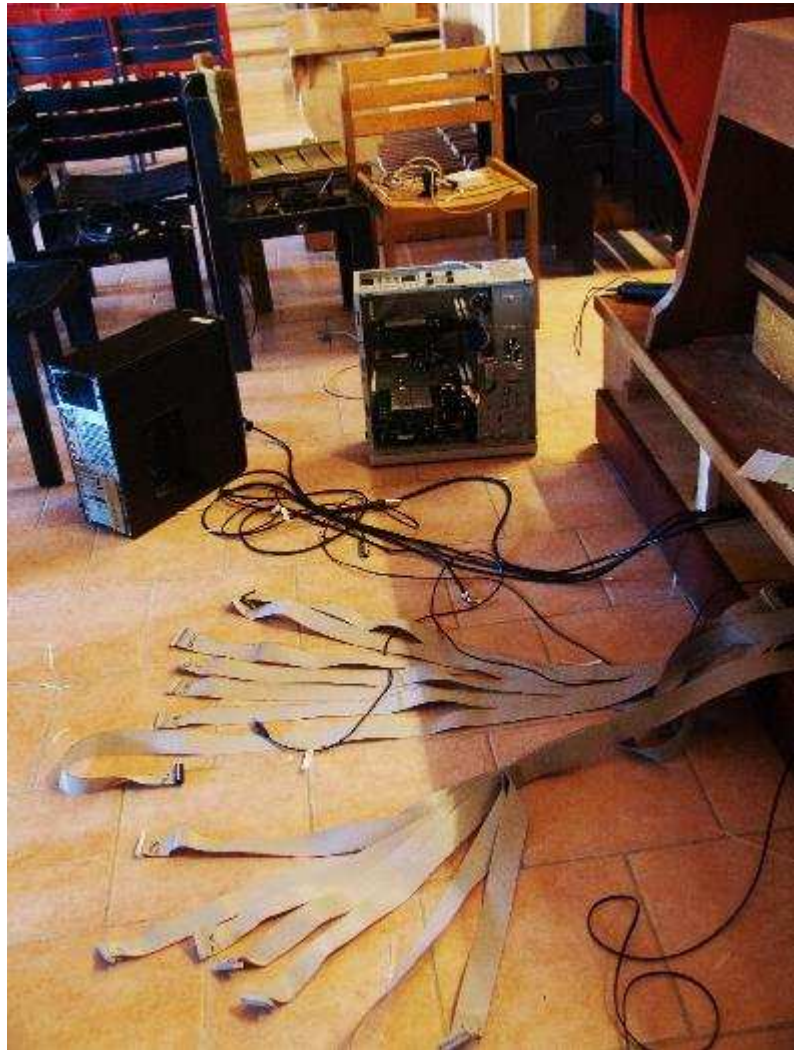
Figure 9: Left side in black housing: the computer for the virtual organ system. In the center: the MIDI electronics in gray housing. Right: the console with the new connection cables.
